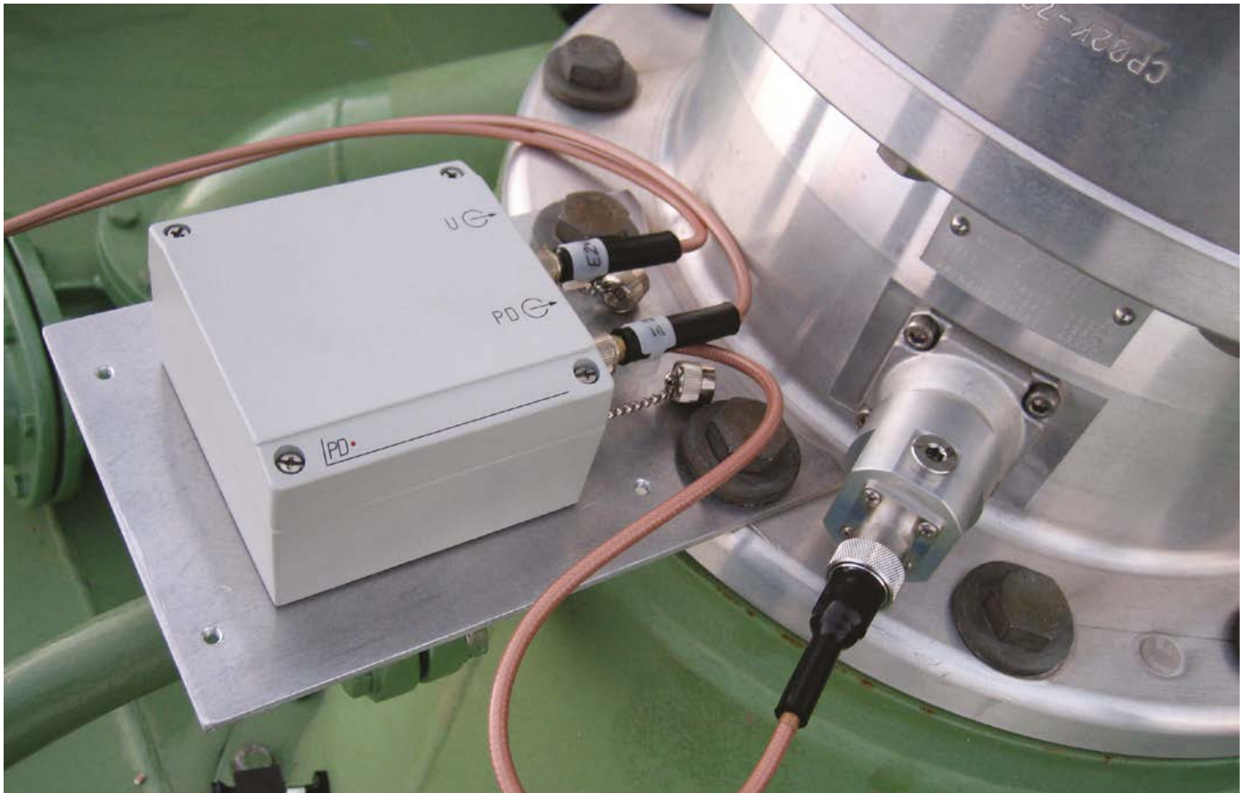
Figure 4. Installed bushing coupling unit and bushing adapter
