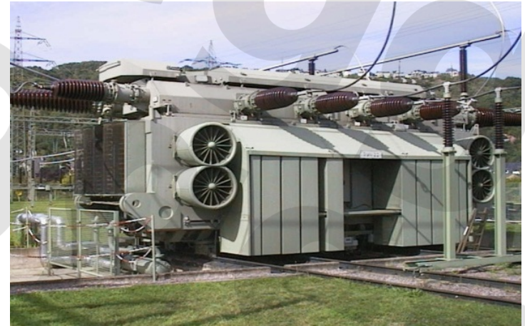
Foto: First PDM installation on a 400kV grid transformer (RWE) 1998
