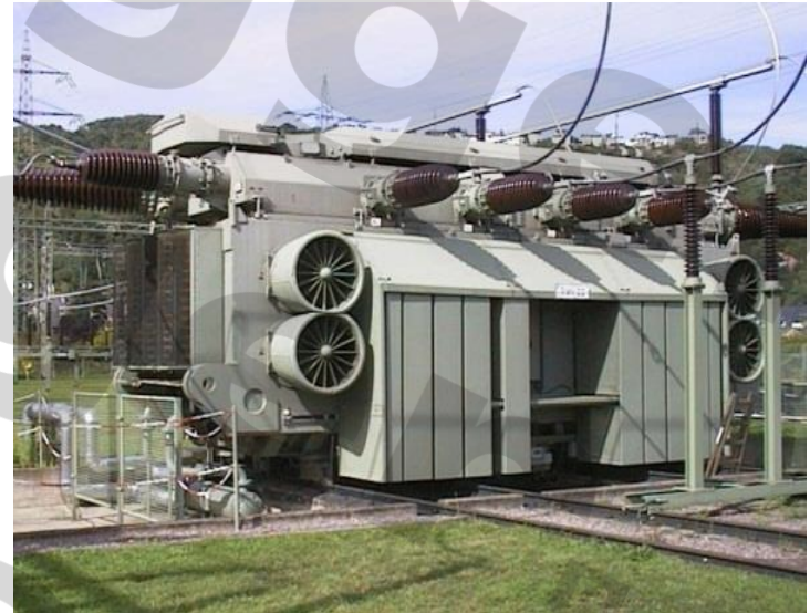
Foto: First PDM installation on a 400kV grid transformer (RWE) 1998
